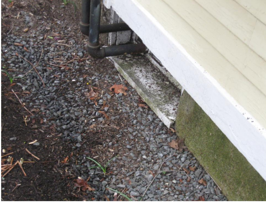
Remove gravel and follow previous instructions for garden area work.
