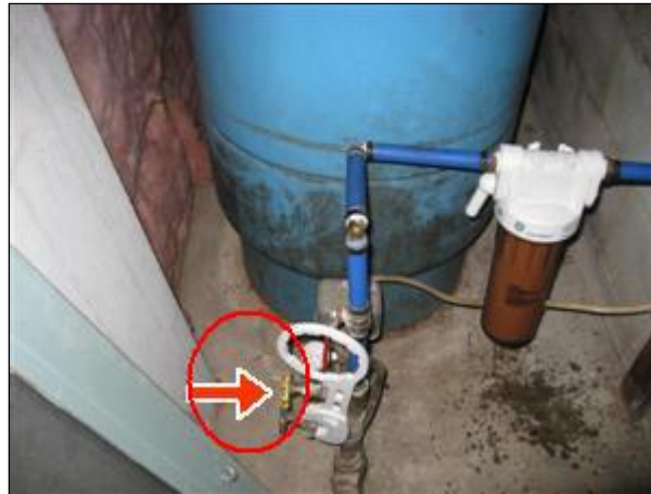
4.3 Picture 1 In basement
