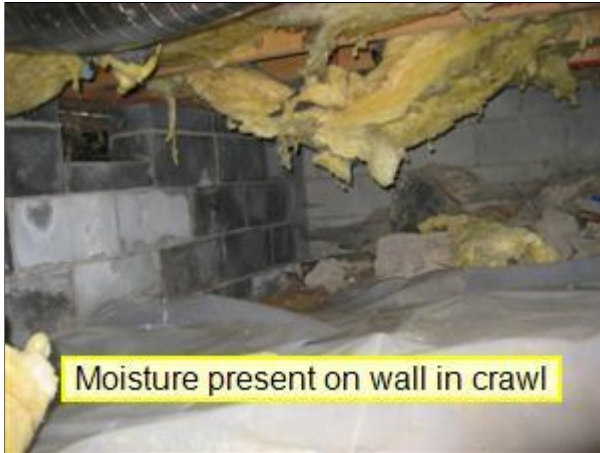
1.0 Picture 5 crawlspace under kitchen
