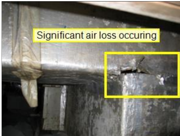
6.3 Picture 4 crawlspace new addition
