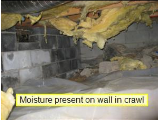
1.0 Picture 5 crawlspace under kitchen
