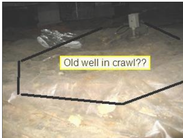
2.6 Picture 2 in crawlspace under new addition
