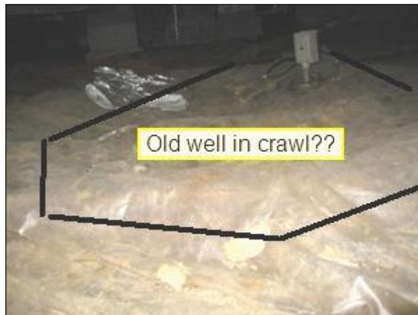
2.6 Picture 2 in crawlspace under new addition
