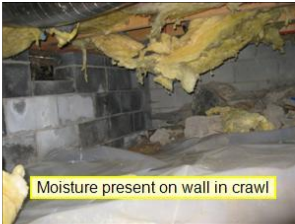
1.0 Picture 5 crawlspace under kitchen
